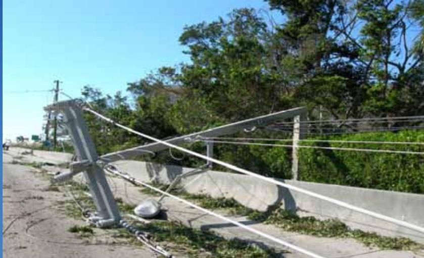
This is a distribution pole, an engineered concrete pole with a very high wind velocity design. It doesn't have a lot of cables hanging on it. Typically a pole is not audited to see what is hanging on it. So many times, poles will fail even though they did not look like they might based on utility records.
